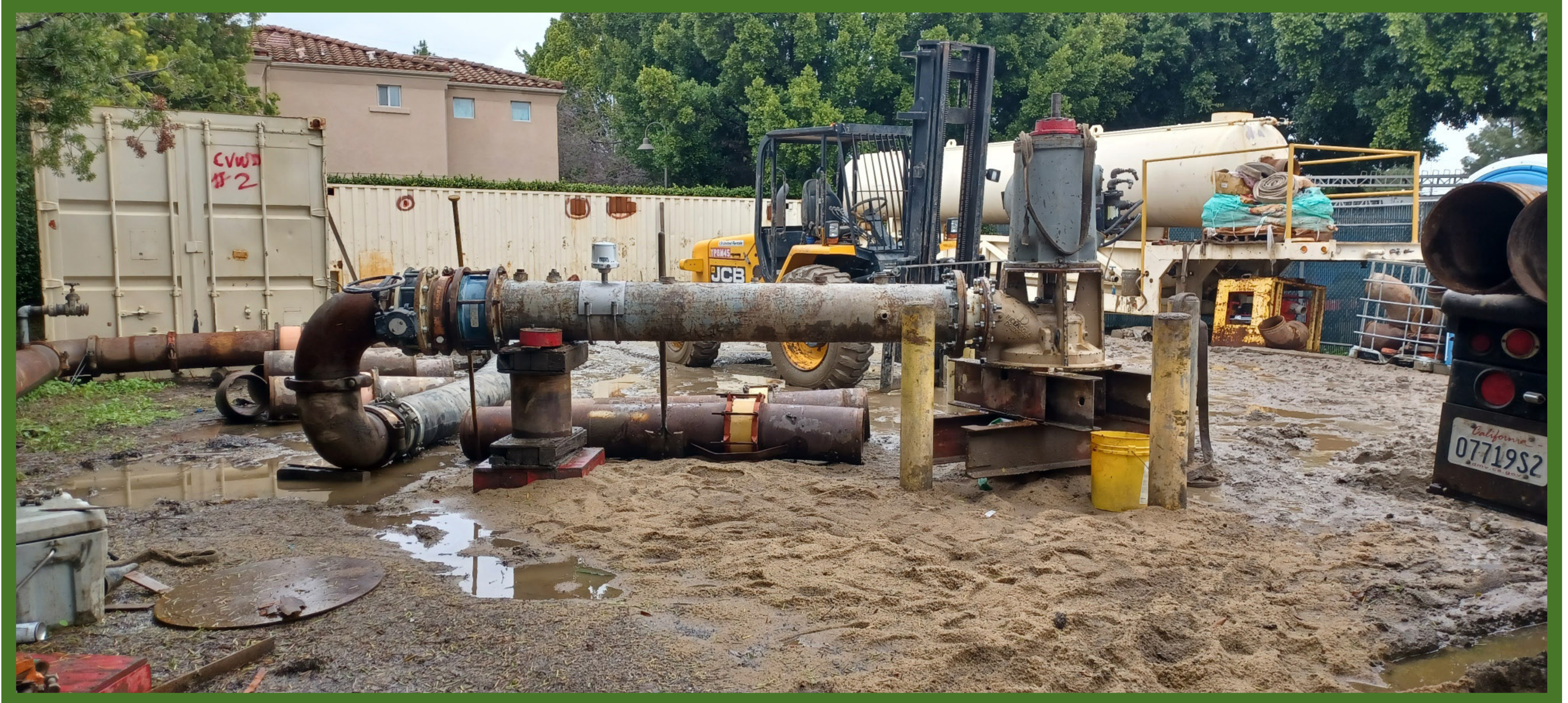
Water pump testing at well
