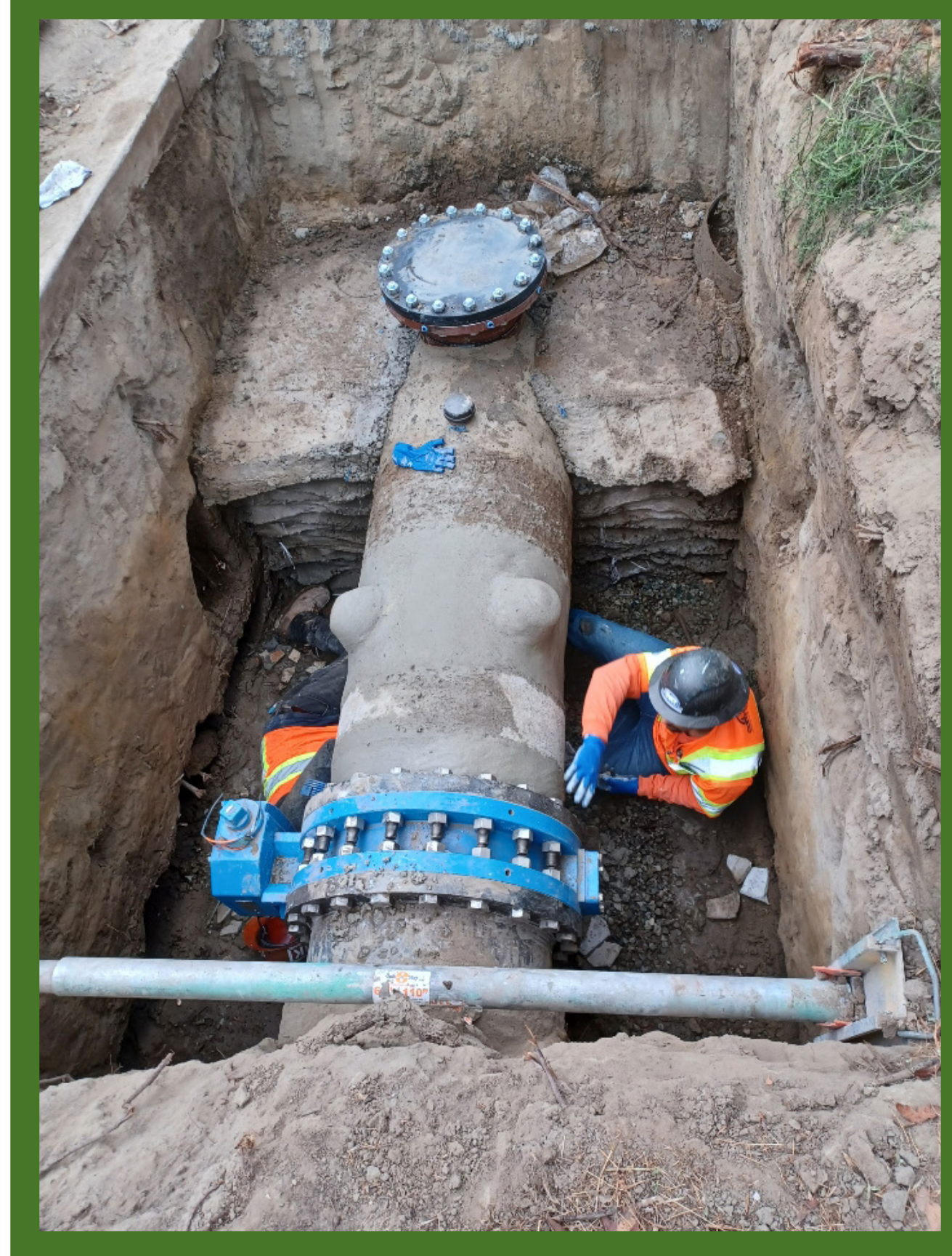
Replacement of water main valves
