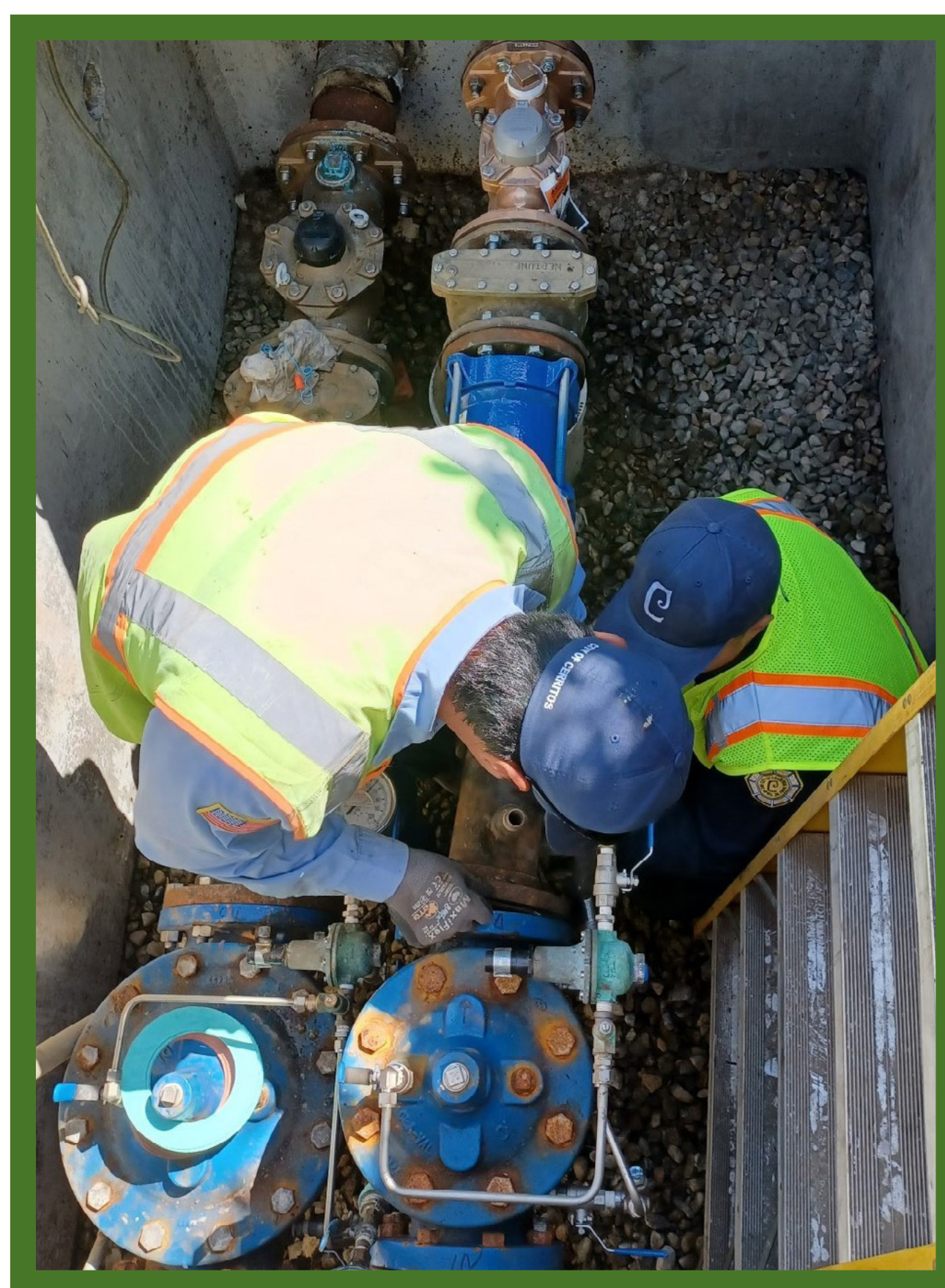
Replacement of 4-inch meter at the Norwalk interconnection
