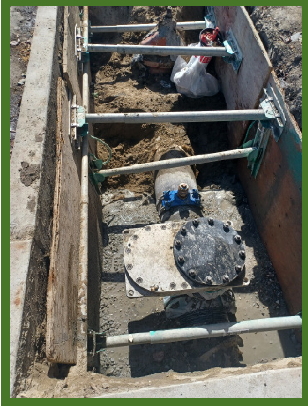
Water meter replacement (interconnection to other cities)
