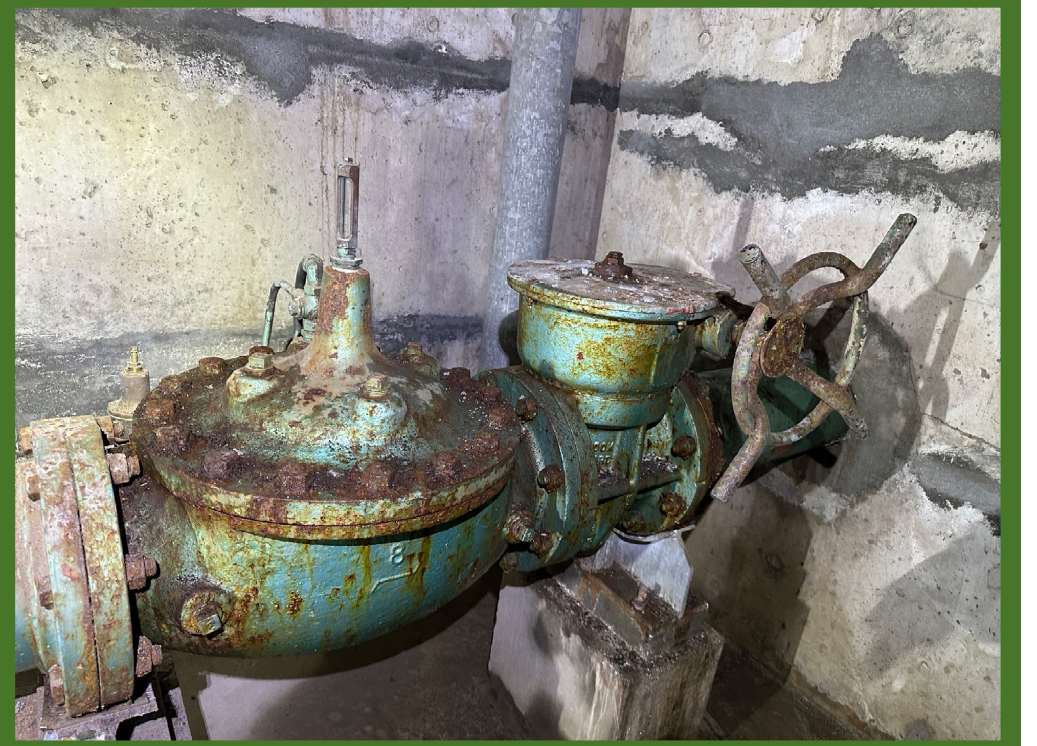
Pressure relief valve in need of replacement (ceased)
