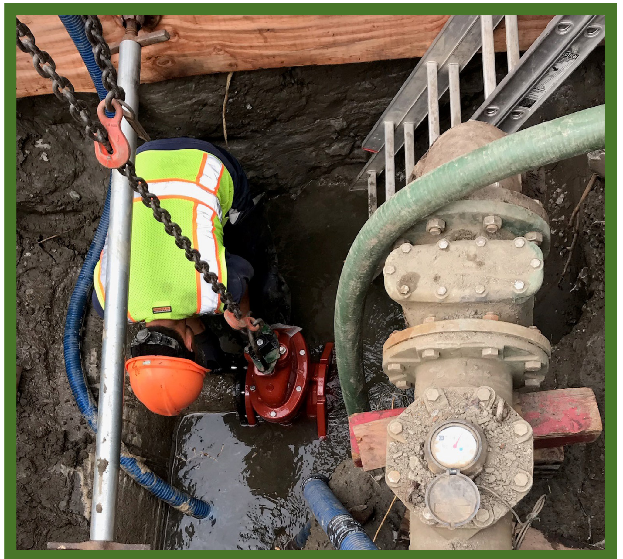
Replacement of 6-inch water valve
