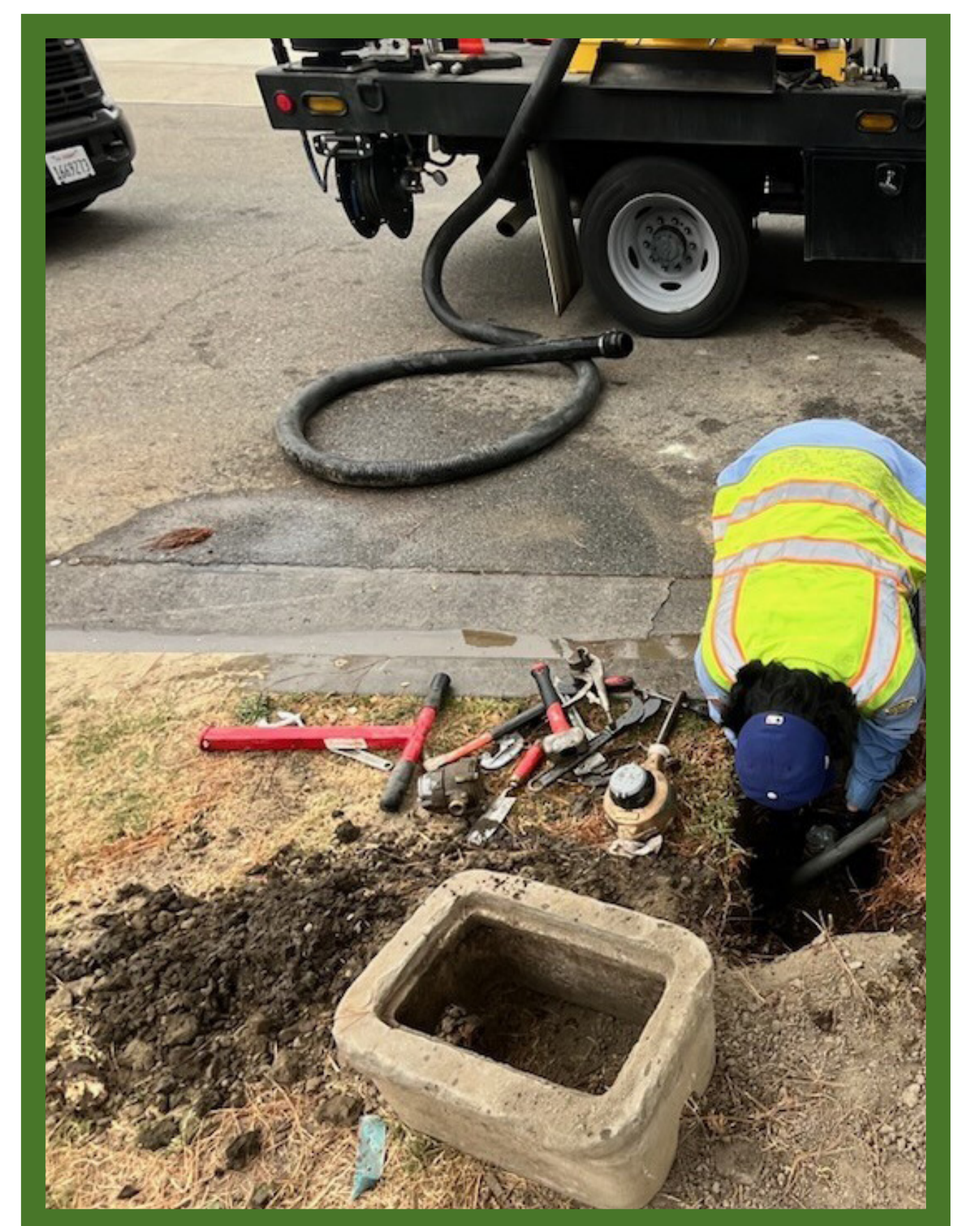
Replacement of meter and angle meter stop at a residence
