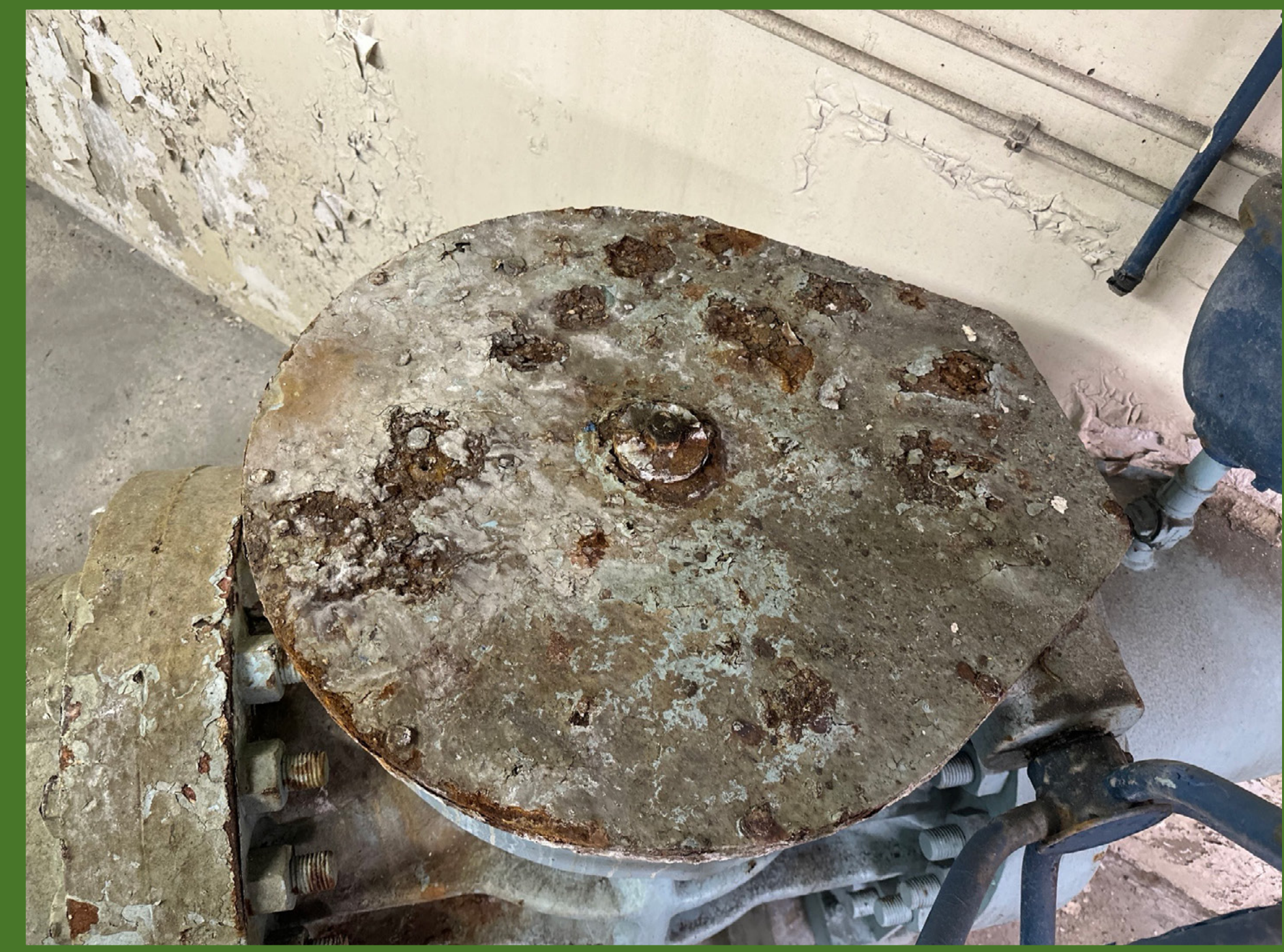
Corroded water shutoff valve in need of replacement
