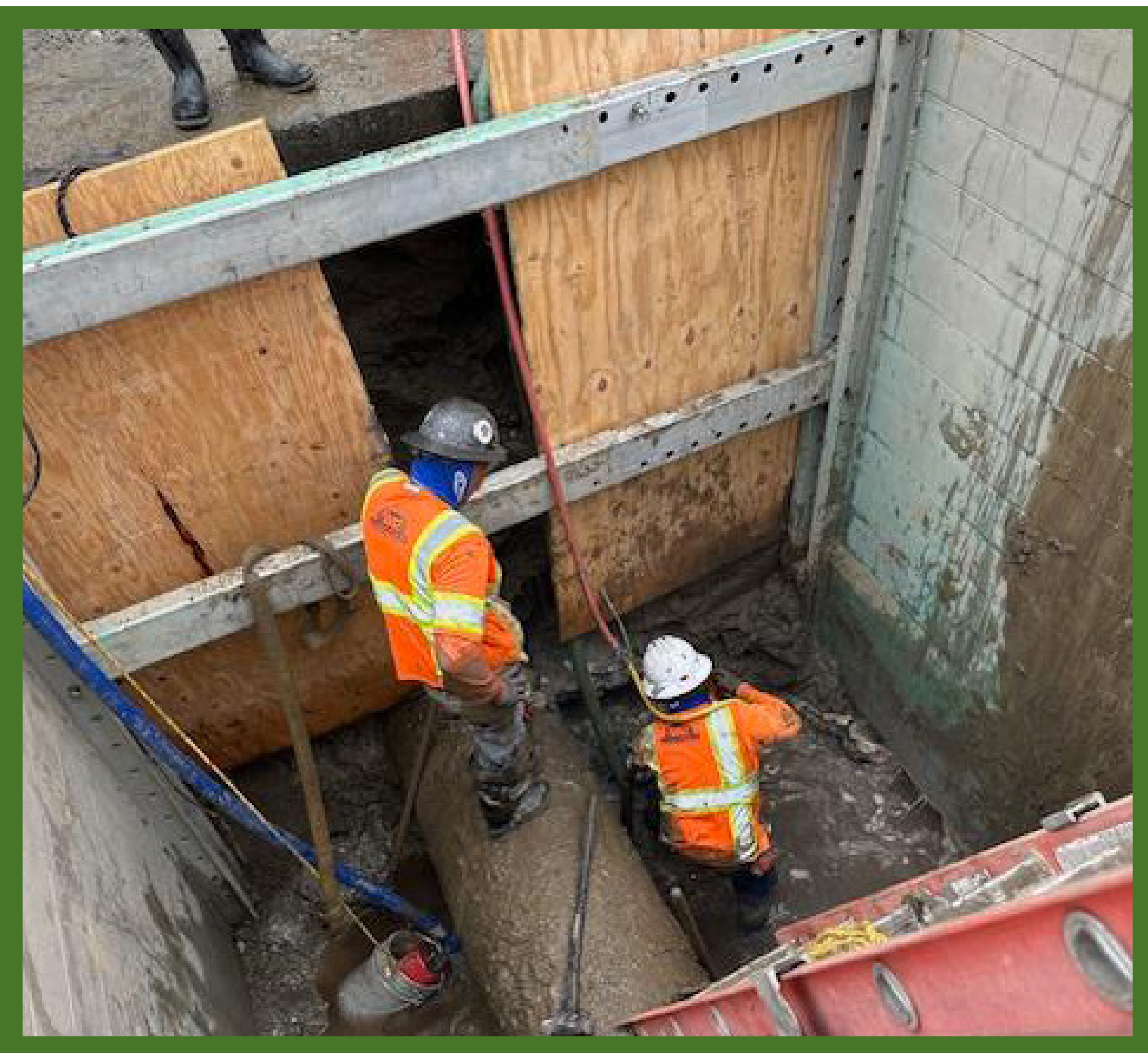
Leak repair of 24-inch transmission line
