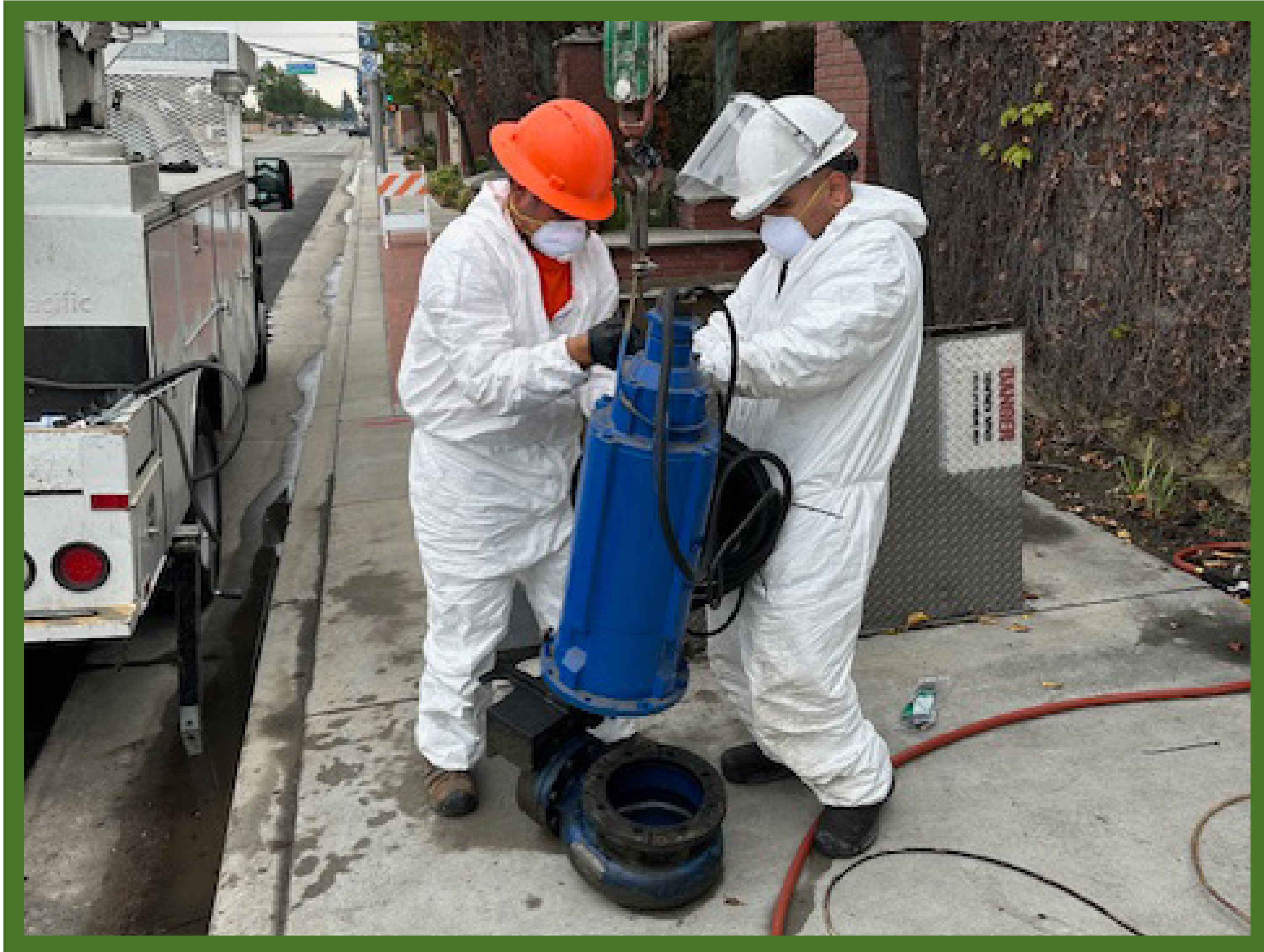
Lift station pump replacement
