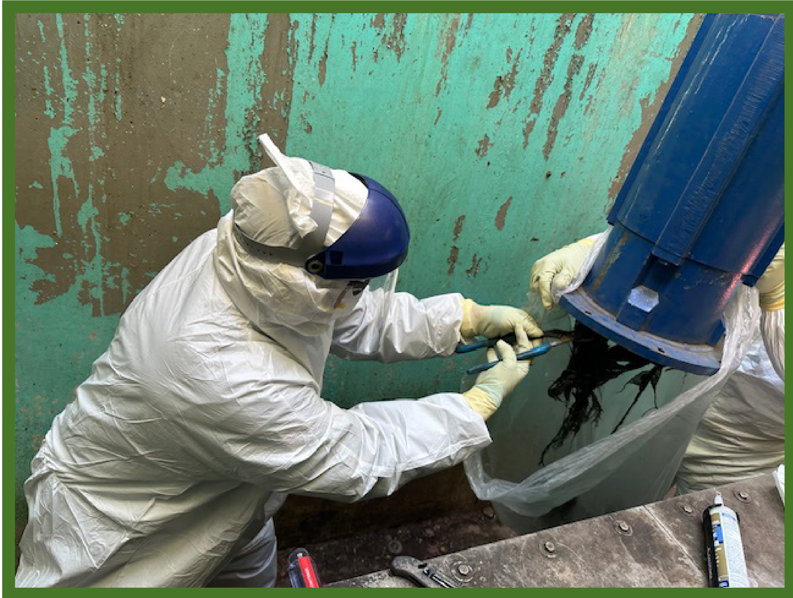
Lift station valve deragging
