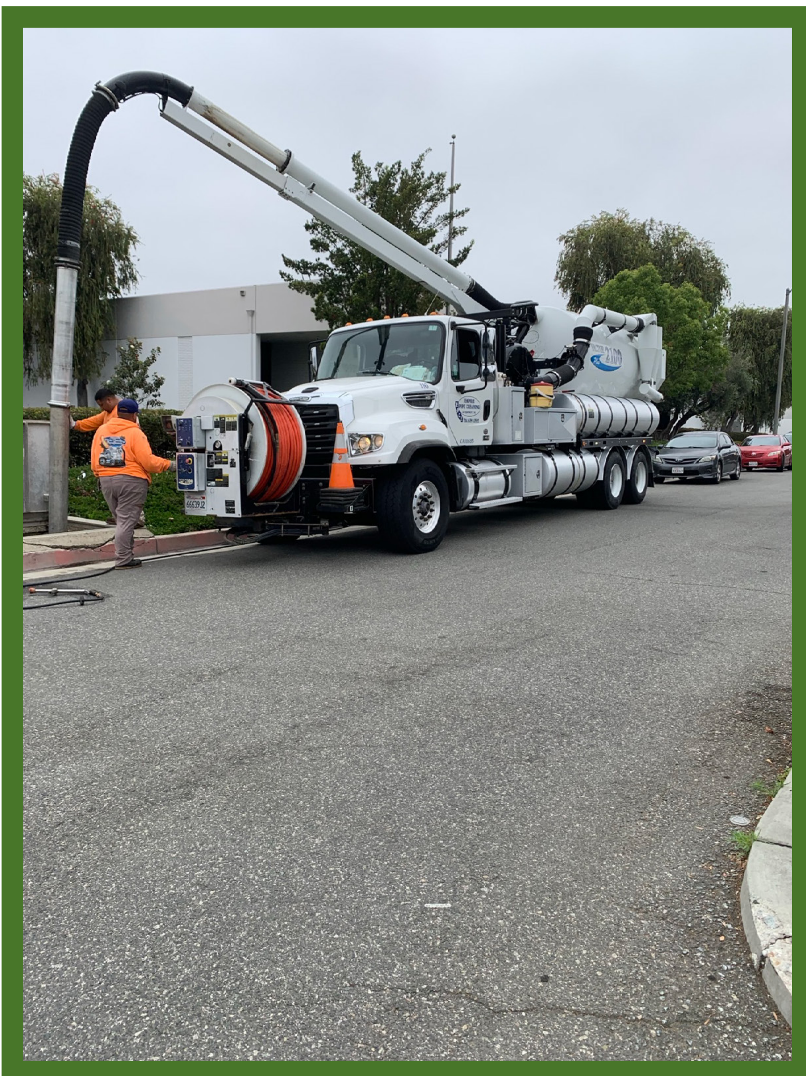
Vactor truck lift station cleaning
