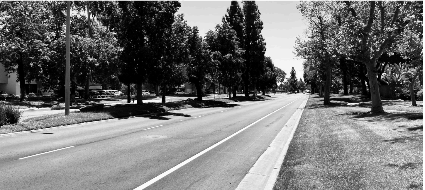
Bloomfield Avenue Street Improvements
